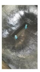
The purpose of the riser pipes is to prevent grit from being drawn up into the septic transfer pump. Any grit that is pumped causes excess wear and damage to the pump and will result in accumulation of grit in downstream tanks like the anaerobic digester.
