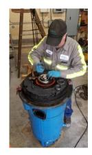
**Septage Acceptance Plant:** The septage holding tank was taken off line to perform a thorough cleaning and grit removal with the VAC truck. While the tank was empty, installation of simple riser pipes was performed.
